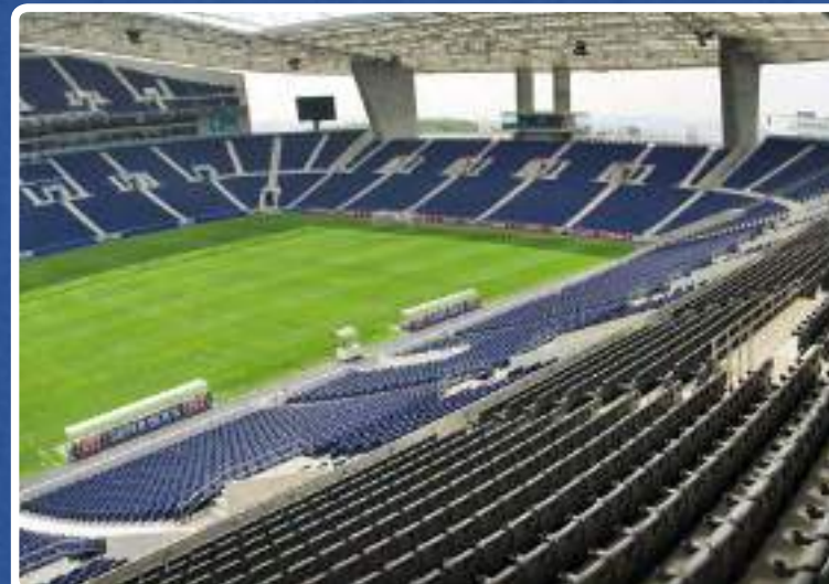
DRAGAO STADIUM, OPORTO, PORTUGAL
