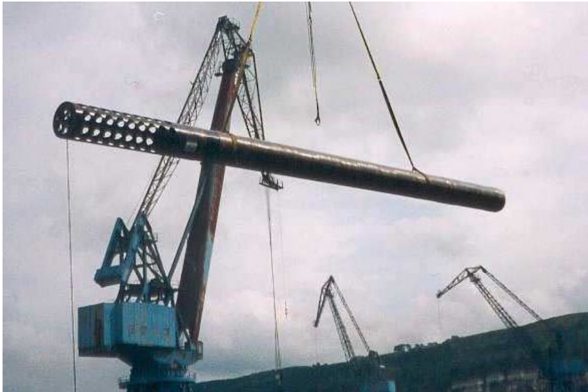
Figure 7. GRE caisson (courtesy of Odebrecht SLP and Ameron BV)
