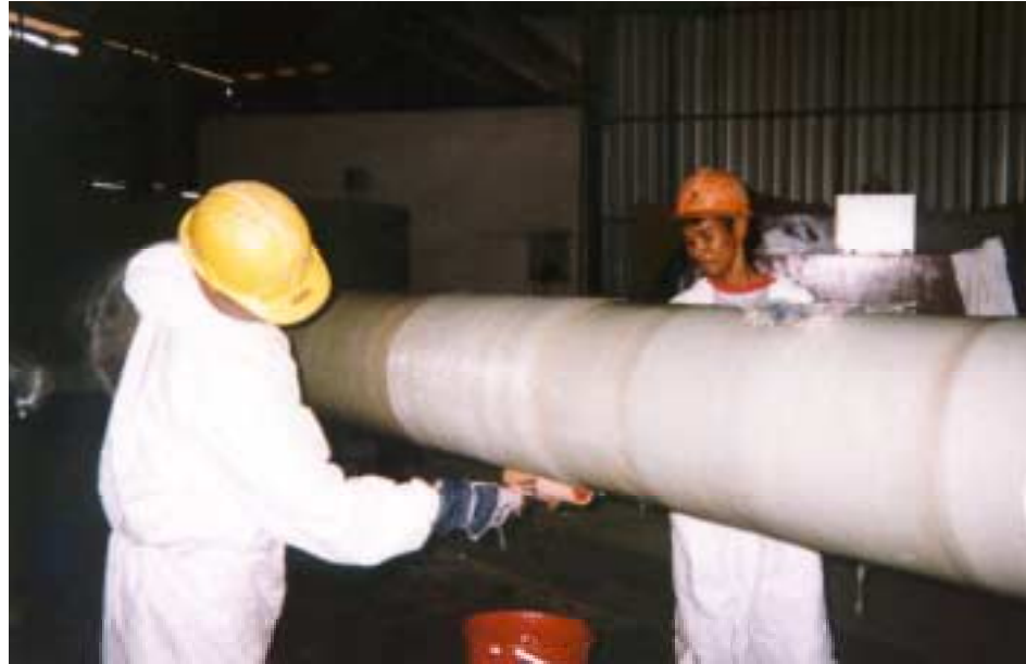
Figure 16. Composite combined corrosion and fire protection being applied to a steel tubular (Vosper Thornycroft (UK) Ltd).
