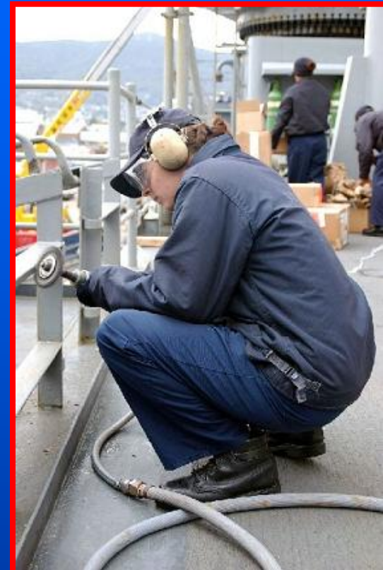
A Sailor uses a Pneumatic Sander to Prepare Metal Handrail for Painting Preservation
