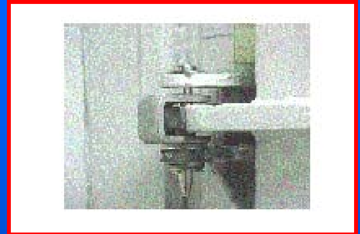
Watertight Door Showing Wear Due to Hinge Misalignment (above) and Corrosion (below)
