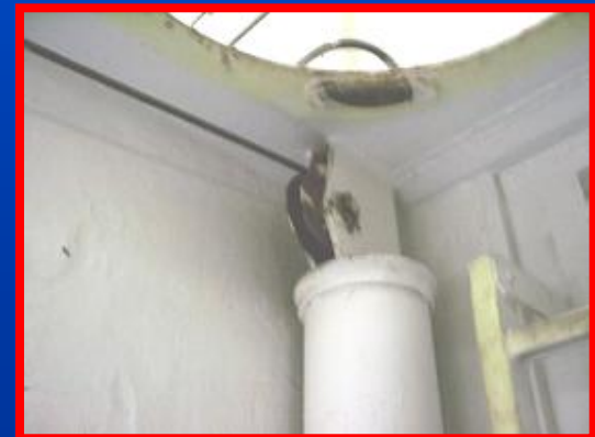
Scuttle Hatch Locking Device (above) and Lifting Assist Mechanism (below) [Ken Brayton, 05P7]
