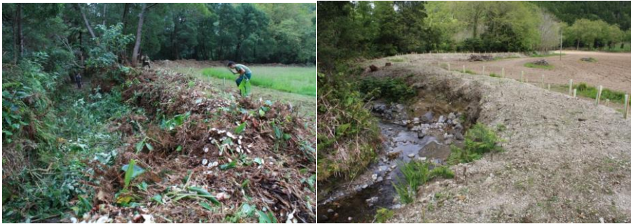
Fig. 26. Rosal's stream bank restoration works, with wicker collection planting. Source: Furnas LandLab photo archive.
