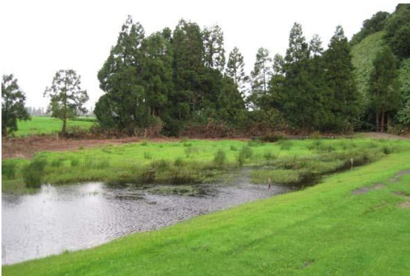
Fig. 11. Wetland created by blocking previous drainages while using stream bed sediments from the installed retention basins. Source: Furnas LandLab photo archive.
