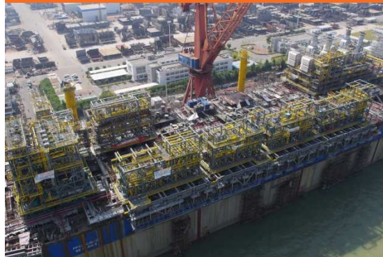
Topside Integration & Commissioning
