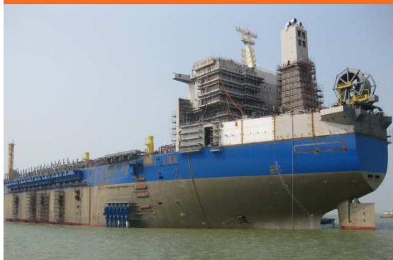
Refurbishment & Conversion of the Hull
