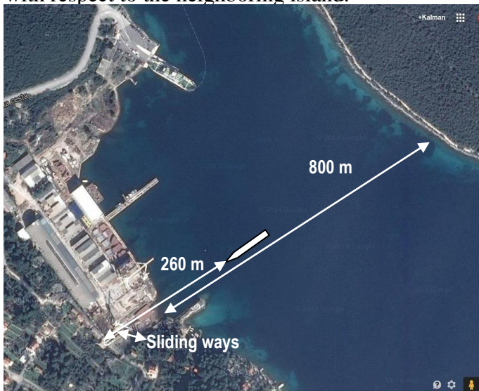
Figure 5. The launching area in Korčula (From Google Maps)
