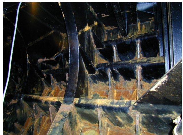
Bow framing in Terry Fox (photo by R. Frederking)
