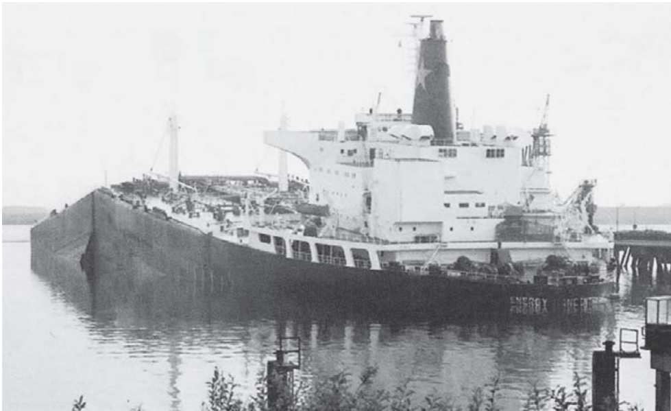
Figure 16.3 The back of the Energy Concentration broke because of poorly executed cargo oil unloading.
