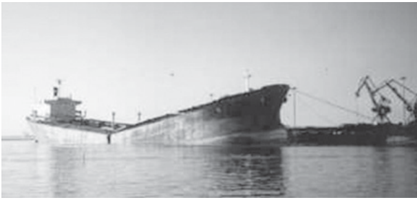
Figure 16.5 The back of the 23-year-old Capesize bulk carrier broke during the unloading of cargo at port.
