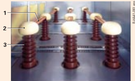
Busbar compartment extending over 3 panels (example) Side view
